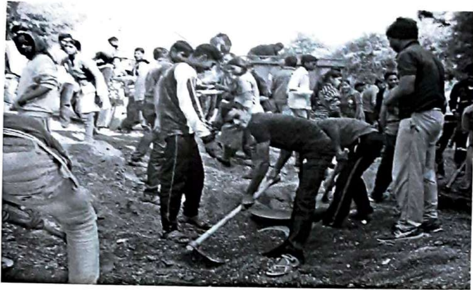
Cleaning of canal for tree plantation
